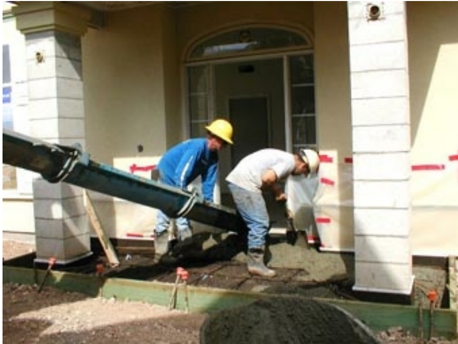
Masons place entry concrete at Apartment 23B.
