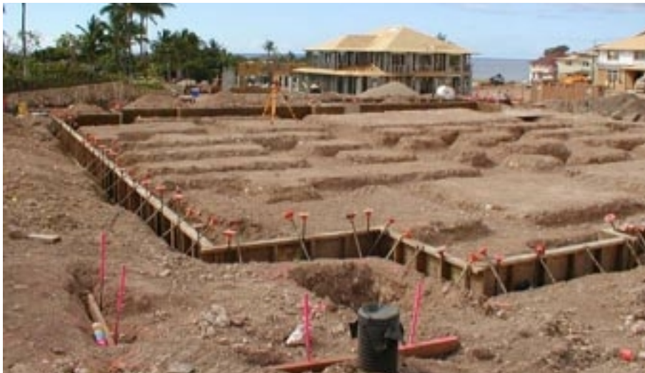
Phase 2 foundation work continues.
