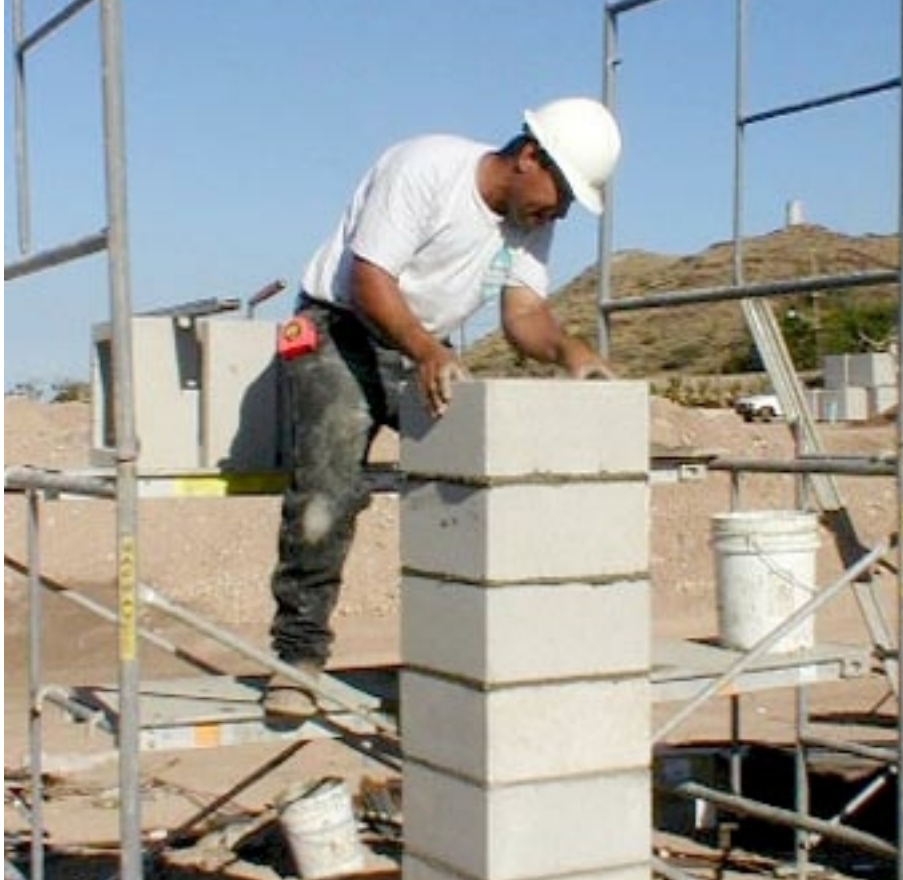
Masonry column is erected at Homesite 7.
