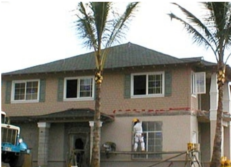
Plaster work in progress at Homesite 24.
