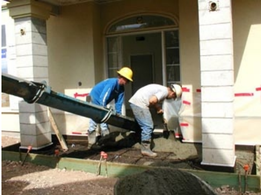
Masons place entry concrete at Apartment 23B.
