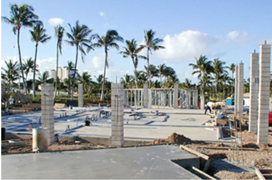
Wall framing begins at Phase 2 Homesite 8.
