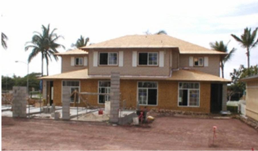
Homesite 1 is ready for exterior paint.
