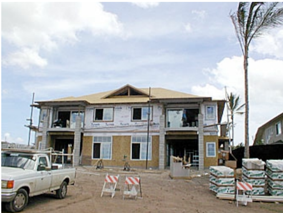
Exterior finishes are installed at Homesite 22.
