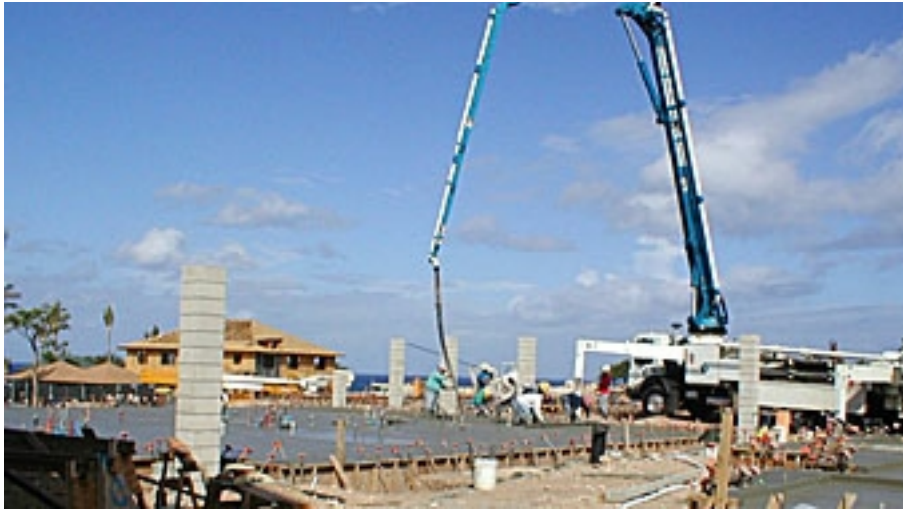
Phase 3 foundations are being placed at Homesite 11.
