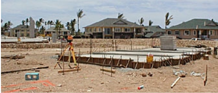
Garage foundation is placed at Homesite 18.
