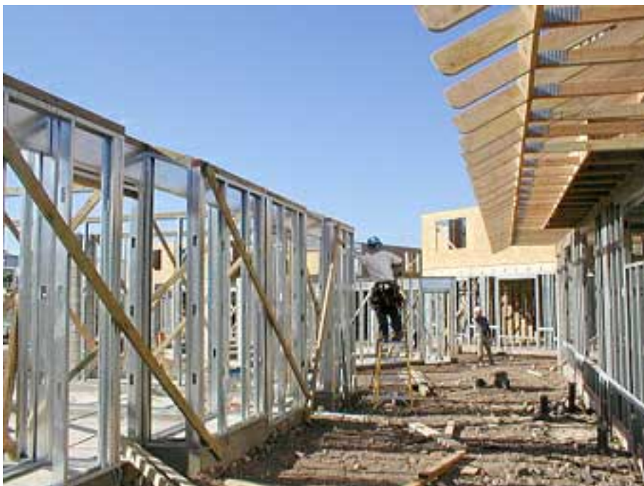
Carpenters continue with framing at home site 23.
