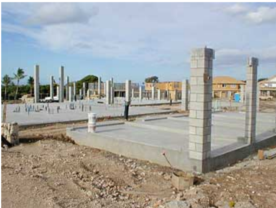
Foundations complete at home sites 28 and 29.
