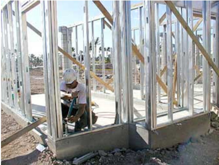
Carpenter installs wind up-lift tie at garage foundation.
