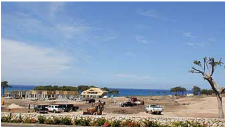
Excavation work begins at home site 1.
