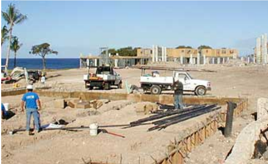
Plumbers install below grade waste lines at home site 4.
