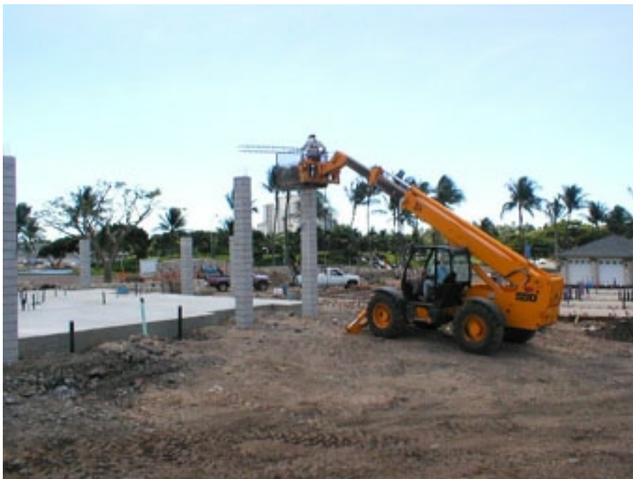
Masons complete block columns at Homesite 4.
