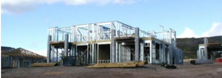
Framing is progressing at Homesite 27.
