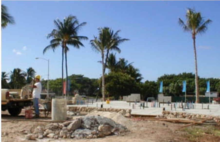
Masons complete foundation at Homesite 1.
