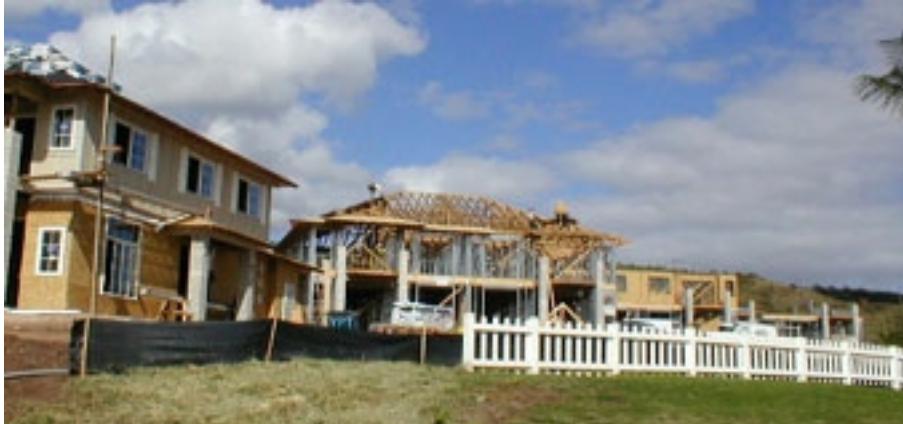
Carpenters install roof trusses at Homesite 27.
