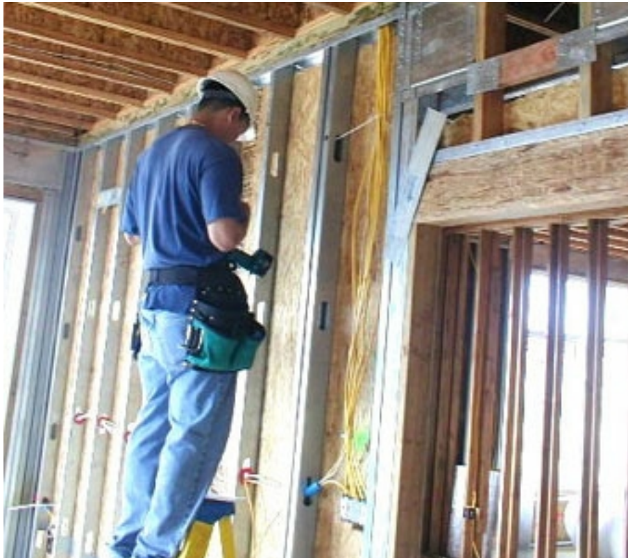
Electrician completes wiring at Homesite 25.
