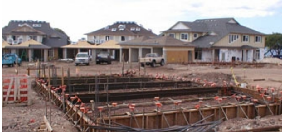
Garage foundation is ready for concrete placement at Homesite 21.
