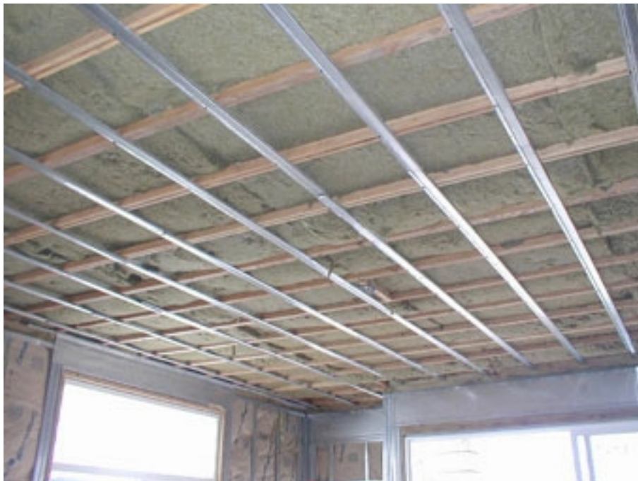
Acoustical sound attenuation system is installed at Homesite 23.
