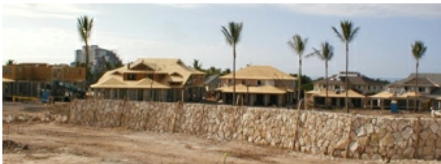
Roofs are framed on Homesite 27,28 and 29.
