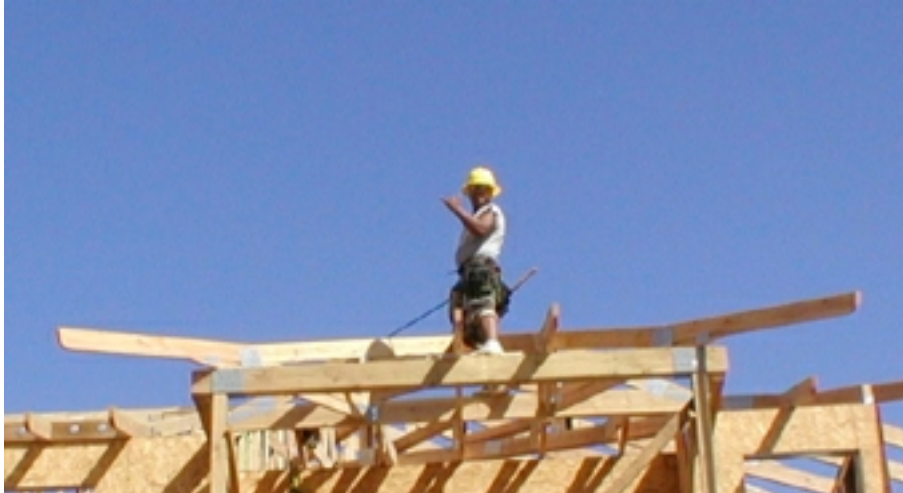
Roof framer gives “Shaka” sign atop Homesite 29.
